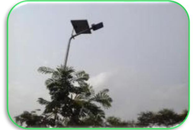
Installation of Solar Street Lights at Dhenkanal and – Paloncha
