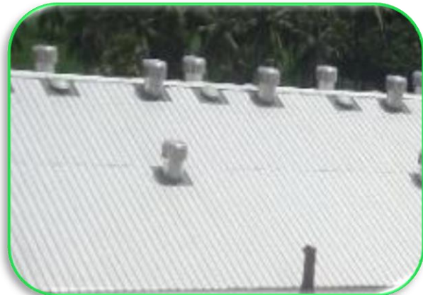
Installation of Turbo Ventilators at Dhenkanal and Samalkot, Andhra Pradesh.
