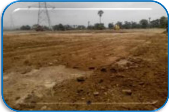
Top Soil Covering
